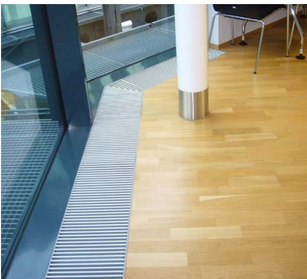
Installation example, with LTG aluminium roller grille
