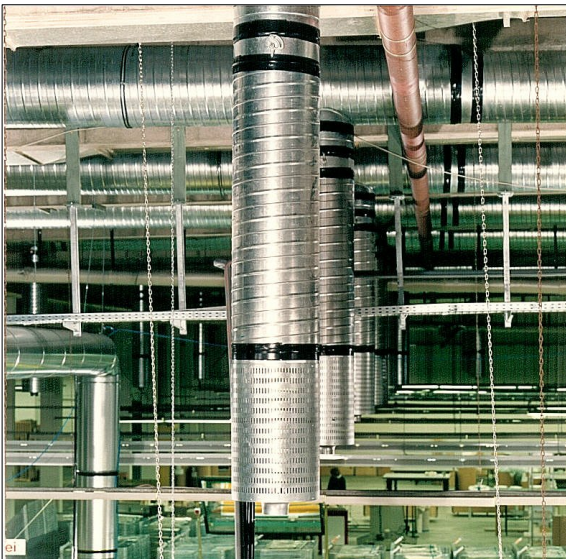
Displacement air diffuser type DLD without nozzle casing, in an industrial hall
