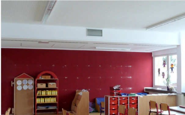
Installation in a ceiling paneling
