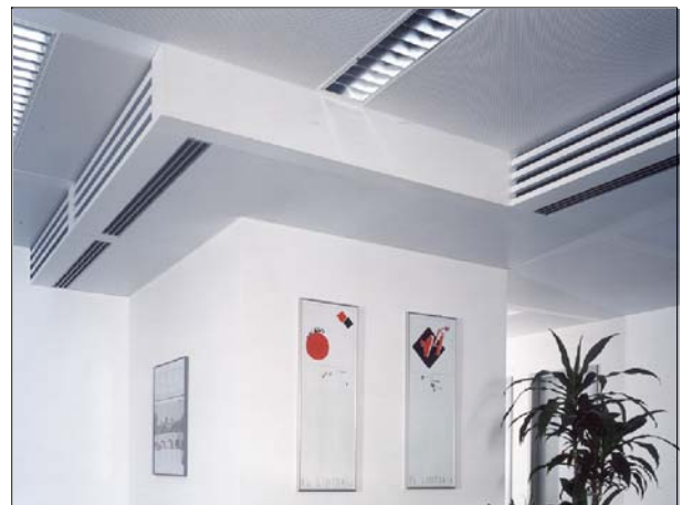
Installation example for LTG air conditioning system Indivent®
